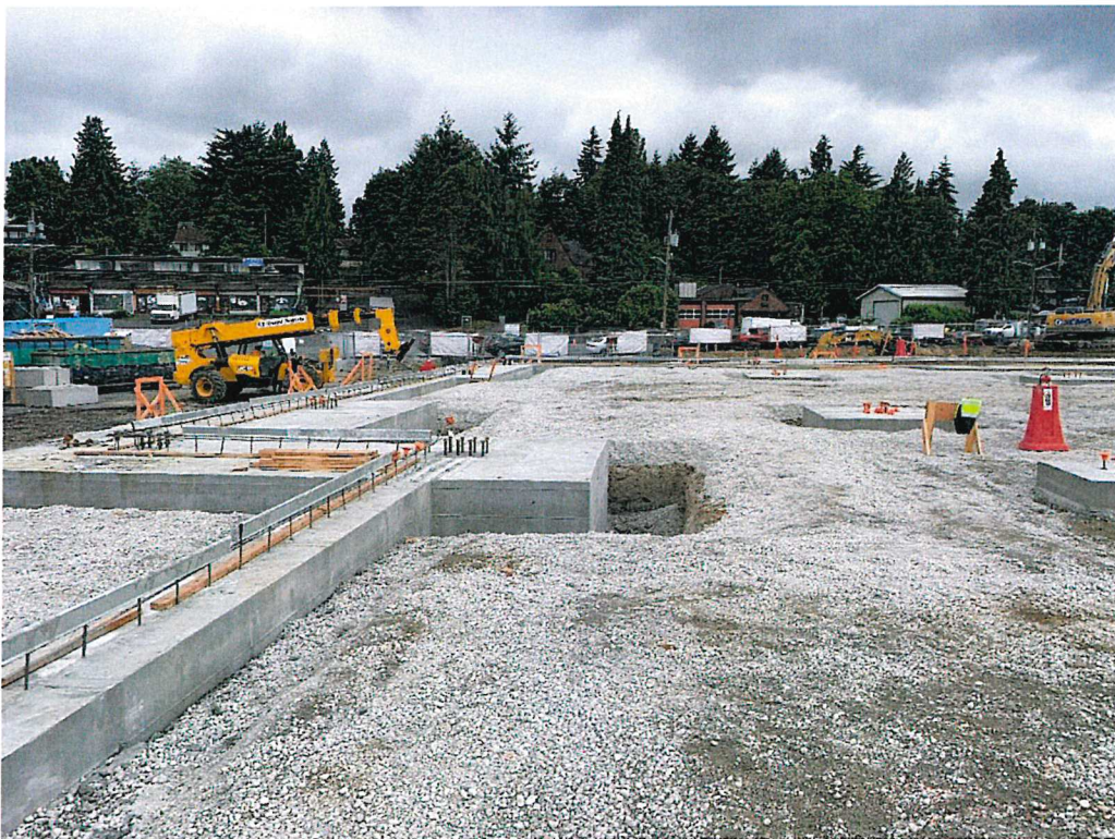
Concrete Footings Poured at South Lot
