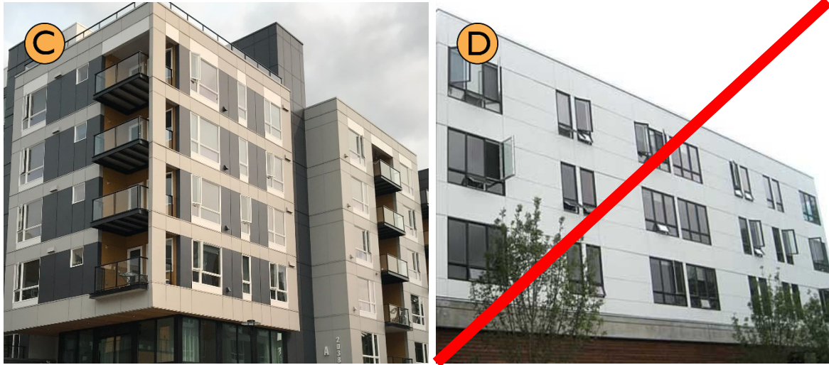
Figure 3.4.D Acceptable and unacceptable cementitious wall board examples.
