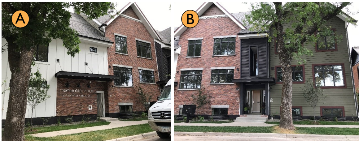
Figure 3.4.D Acceptable and unacceptable cementitious wall board examples.
